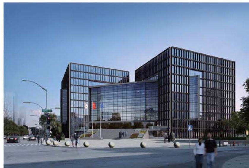
新总部 New Headquarter (under construction)
